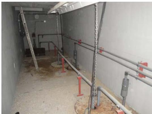
**Figure 1.** Tun system with tanks in a concrete bed
