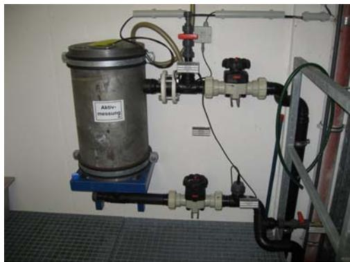
Figure 7. Fast on-line control measurement in the release line (flow through measurement)
